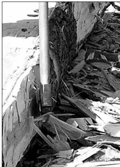
Fig. 5 The beams are all made smooth with an axe. ■
