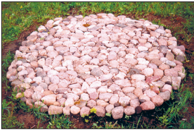
Fig. 1 Bed of the stove, made from small granite stones. ■
