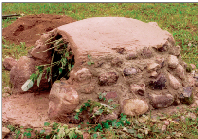
Fig. 4 The finished construction. ■
