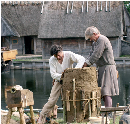
■ Fig. 6 The reconstructions department from Aarhus University is making an oven to cast a replica of the Loshult gun in lost wax technique
